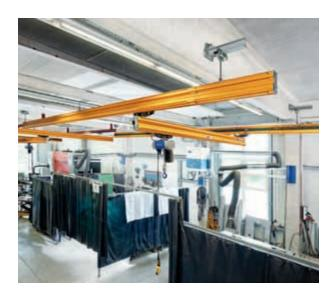
Support consoles are fastened laterally on the building trusses. Heavy-duty anchor bolts are used in the fastening. There are anchor bolts for concrete as well as wooden trusses, with varying projection lengths.
