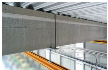
The threaded rods at the side are variable in length and enable even large truss heights to be used. Depending on the ceiling construction, embracing brackets can also be mounted on the ceilings on top of the building trusses.
